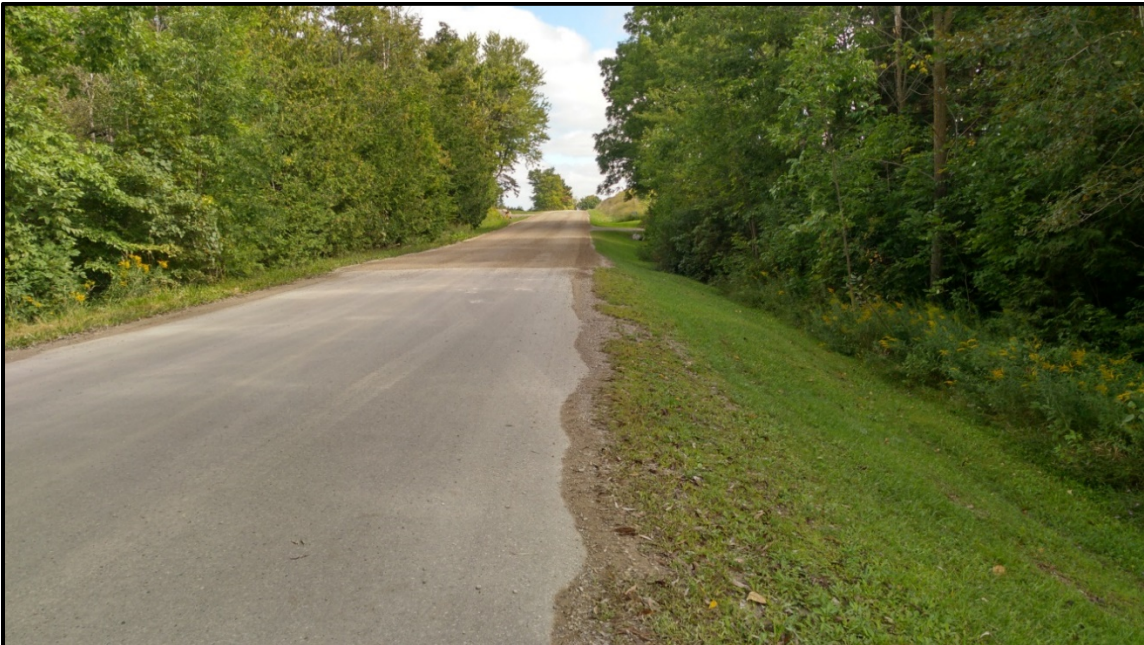
Image 8: Disturbed ROW in in Northwest Portion of Project Area (looking northeast)
