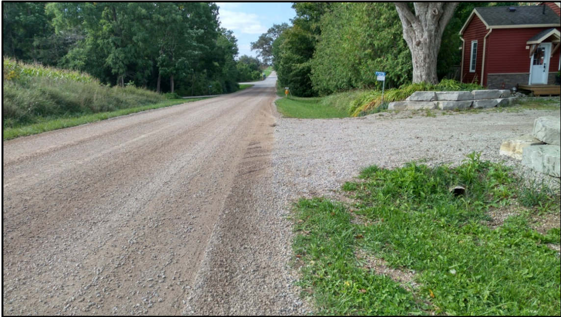
Image 7: Disturbed ROW in in Northwest Portion of Project Area (looking southwest)
