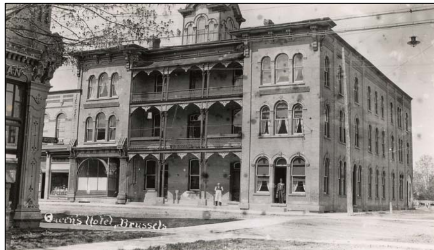
The main façade of the Queen's Hotel with its two projecting wings and handsome piazza, the centre being topped by a lofty and highly ornamental rectangular tower, surmounted by a cupola whose top is protected by a handsome iron railing.
