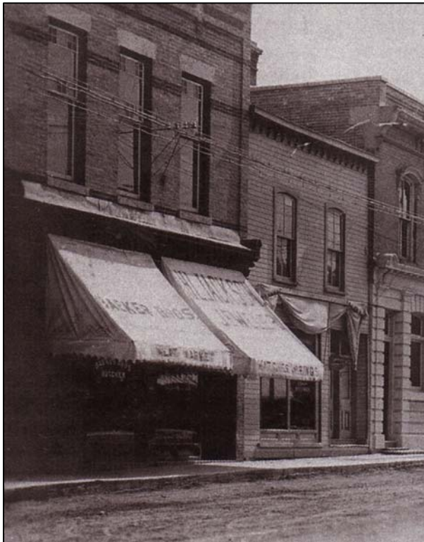
The Blashill Block with Baeker Bros. Meat Market and HL Jackson's jewellery store. The Gerry Building with Wright's express office is to the south, and the Leckie Block with its new front to the Standard Bank.
