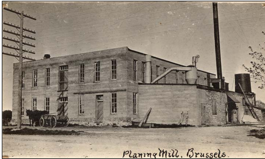
Williams Livery was converted into George Edwards Planing Mill in 1894. An engine house was built at the rear of the shops to house a 16-horse-power boiler and engine. Advertisements from Brussels Post – Right: March 16, 1894; below: 1897.
