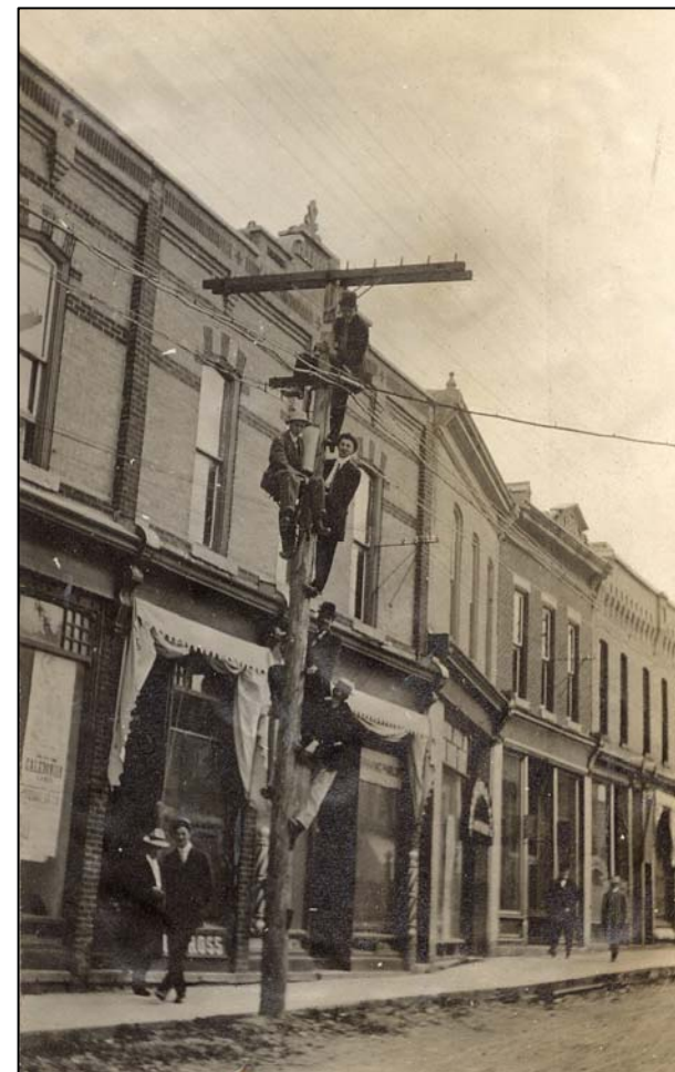
Men up a pole in front of the Leckie Block 2. "Ross" marks the north store in the Leckie Block. DC Ross may have moved here after his partnership with Ferguson dissolved in 1909. Barbers poles mark Elliott's shop in the south store. Note the angle of the addition to the south of Leckie Block 2 made in 1900. John Walker was the tenant of the new store. The Drewe Block is next and then the Shiel Block.
