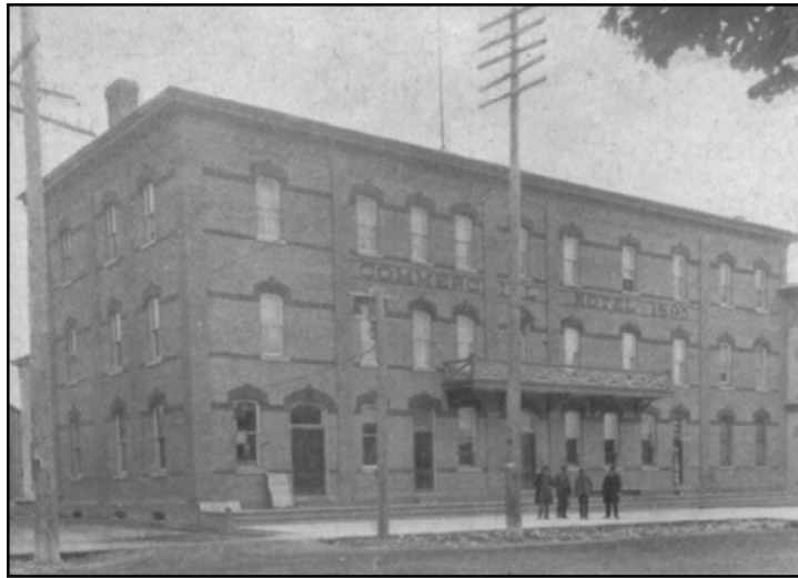
The Commercial Hotel as pictured in A Souvenir of Seaforth published in 1900. You can clearly see the horizontal bands linking the window arches and sills of each storey. Pilasters mark off four sections vertically across the facade. Note that there are four separate entrances. Ads, from top right: Huron Expositor , February 20, 1891; Seaforth Sun , June 8, 1883; Huron Expositor , March 11, 1898.
