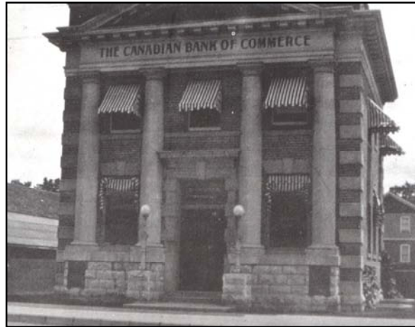
Here, the Canadian Bank of Commerce is dressed with striped awnings on all the windows.
