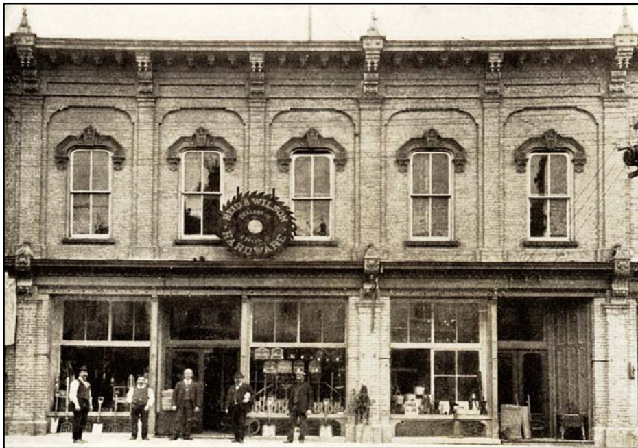
Reid & Wilson's Hardware as it was in 1900. Note that the architectural details of the original have been beautifully recreated so that the existing building looks much as it once did.
