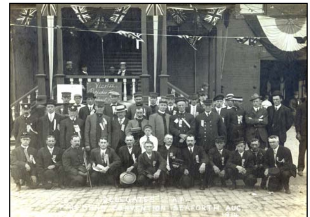
In this photograph taken in 1914 you can see the original location of stairway leading to the second floor.
