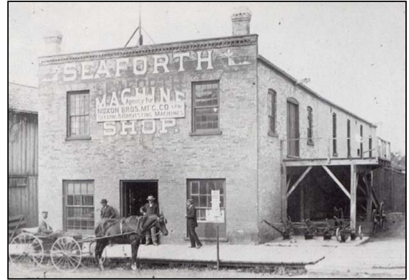
This building housed McIntosh & Morrison's Carriage Shop in the 1870s and then O.C. Wilson's agricultural implements business. Advertisement below, The Huron Expositor , February 20, 1891; at bottom left, April 11, 1884.
