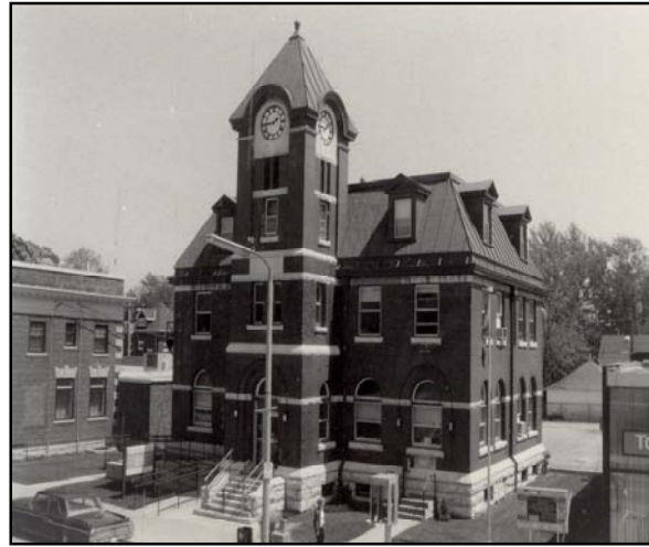
Note the rusticated stone foundation and the use of the white stone in the banding and window sills.
