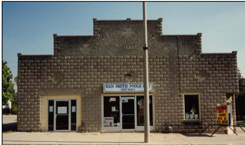
Ken Smith Pools was in business in the Gallop Building in the early 1990s. The photograph clearly shows the boomtown or corbie-stepped roof.
