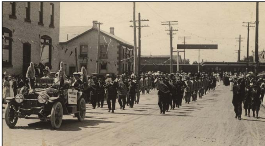
This photograph of the 1914 Old Boys Reunion parade shows the Grip House in the background at left. By then it was Duncan's Legging & Shoe Factory.
