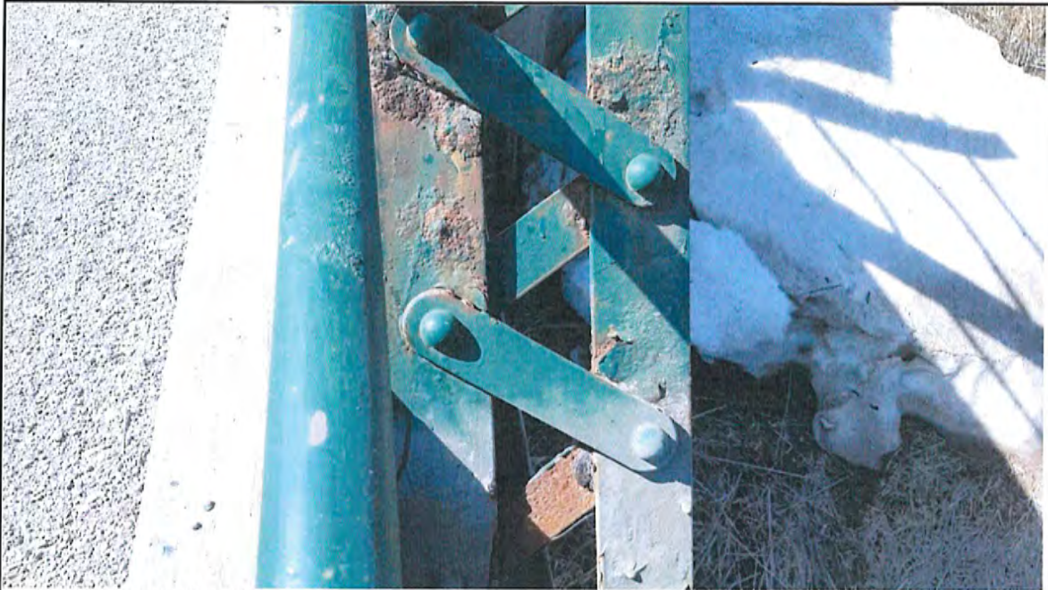
Diagonal - West Truss
