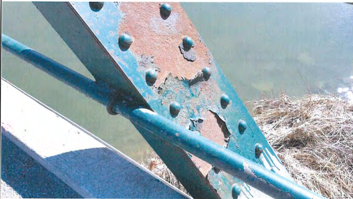
Top Chord at Southeast Corner
