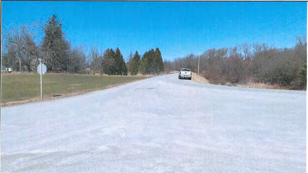
Intersection South of Truss - Facing West
