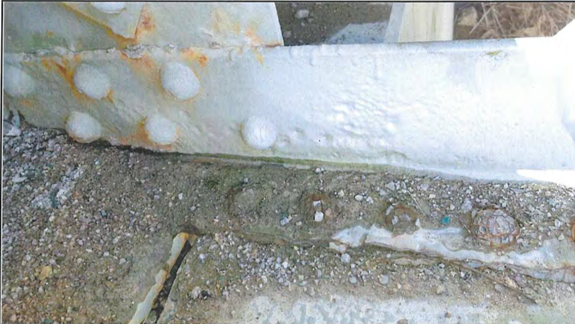
Southeast Bearing Connection
