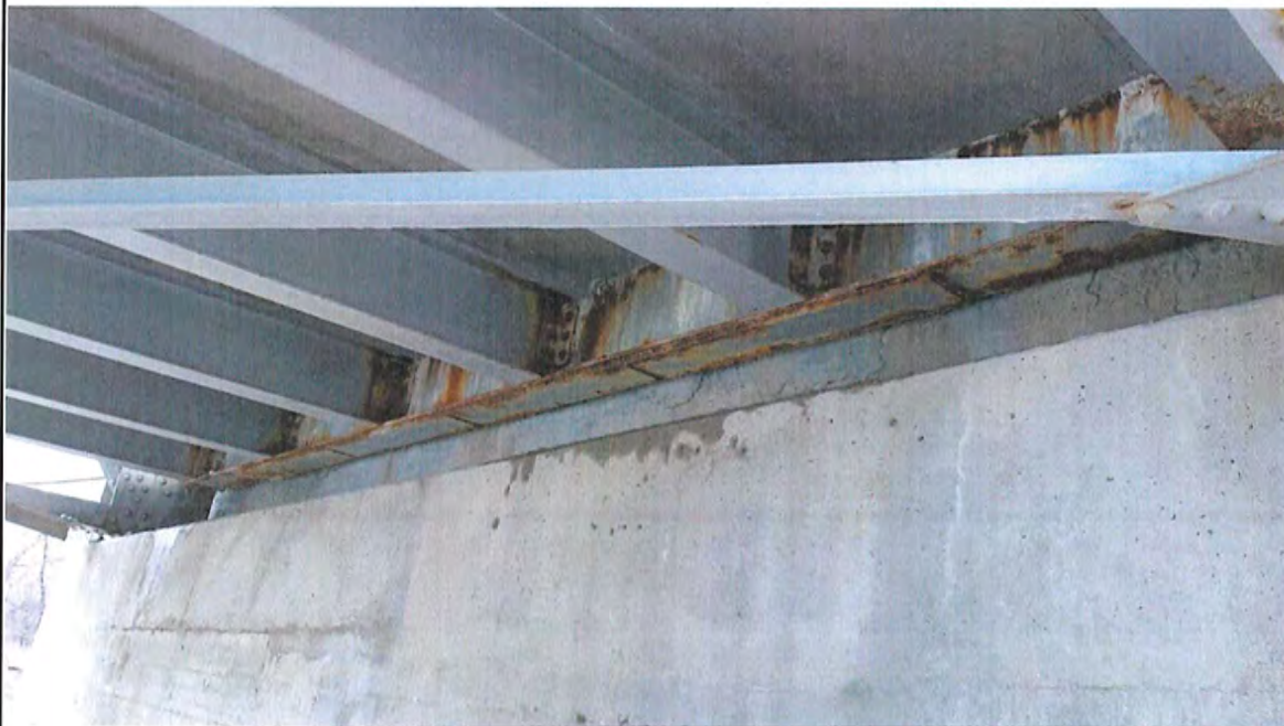
South Cross Beam
