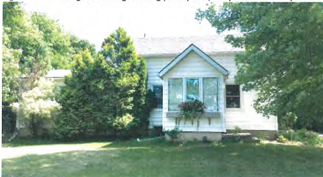
Figure 4: Image of Existing Dwelling (front porch/entry to be removed)
