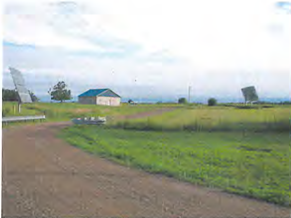
10 kw Solar Trackers at Seaforth Water Plant
