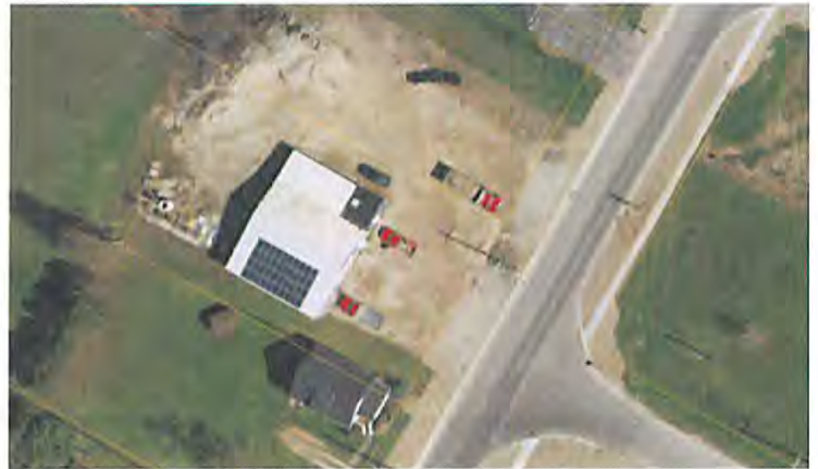
10 kw Rooftop Solar at Brussels Public Works Building
